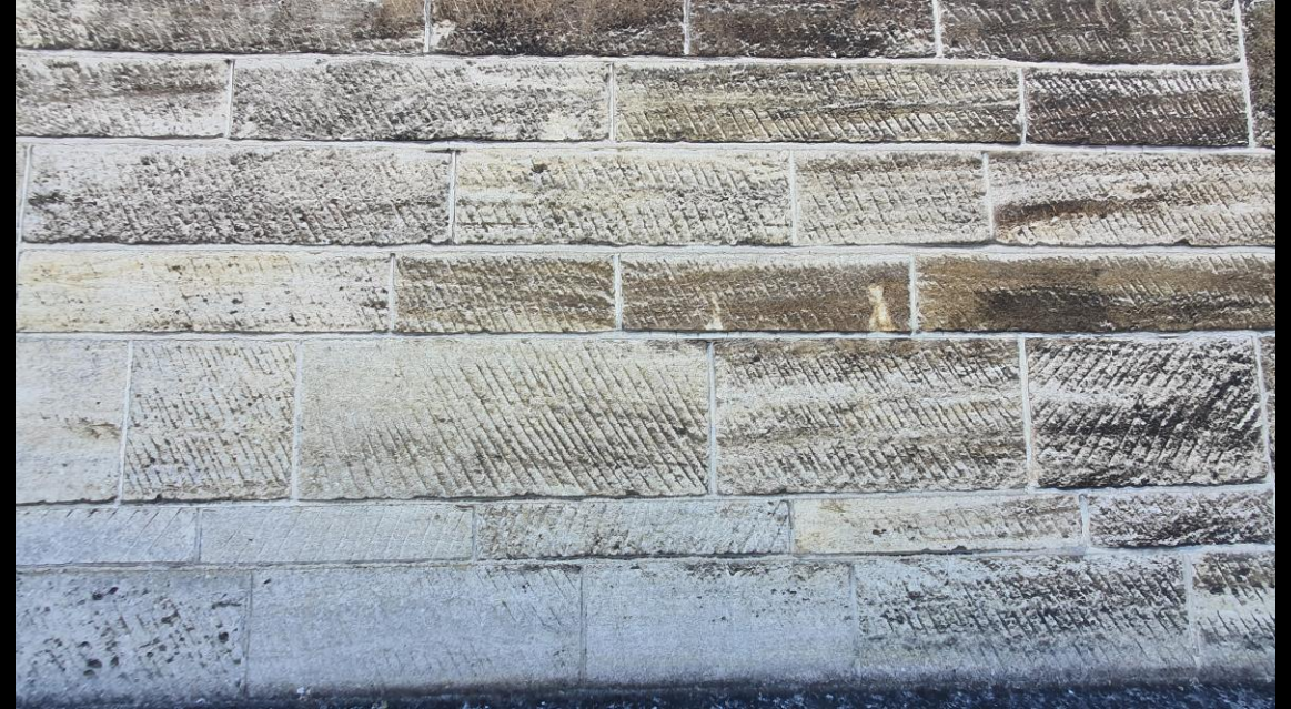
Boasted or droved finish: parallel lines cut with a wide-edged chisel called a 'boaster'.
