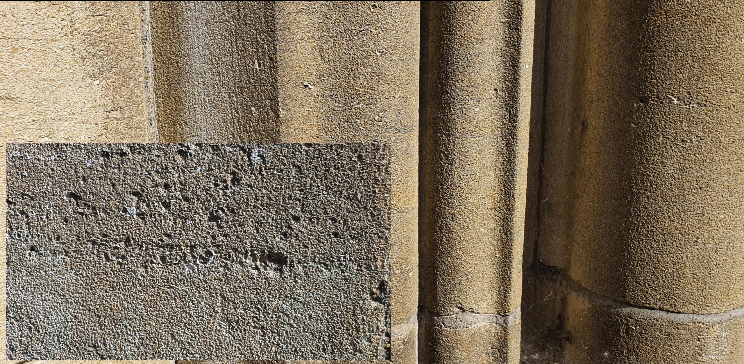
St John's Church, Greenhill: Stone detail - 2 Showing texture and shell debris
